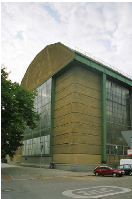
depicted item: Hutten-, corner Berlichingensstr., source: Winfried Brenne Architekten, date: August 2006
