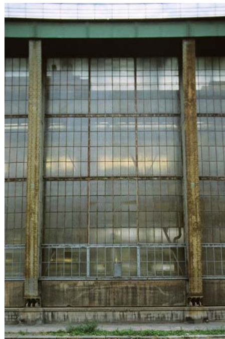
depicted item: detail façade Berlichingensstr., source: Winfried Brenne Architekten, date: August 2006
