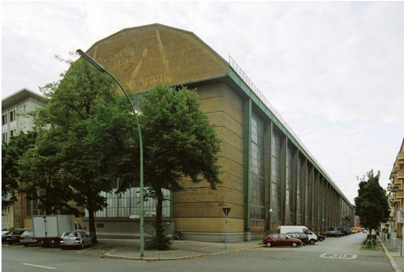
depicted item: Hutten-, corner Berlichingensstr., source: Winfried Brenne Architekten, date: August 2006
