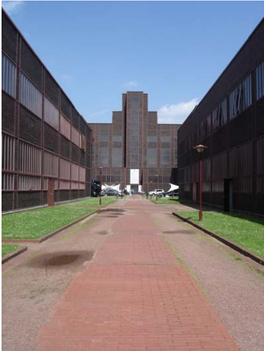
depicted item: view to boiler house source: docomomo Germany, Foto: Borgert date: June 2008
