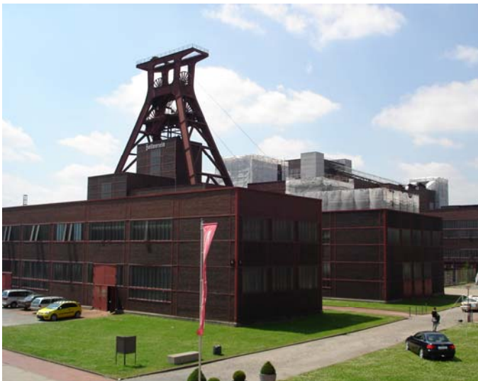
depicted item: Zollverein Pit Shaft XII with workshop buildings source: docomomo Germany, Foto: Ulrich Borgert date: June 2008
