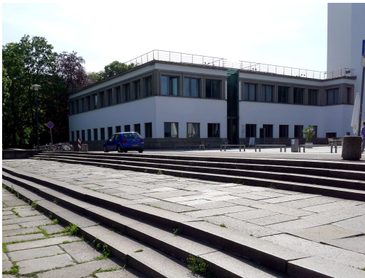
Picture 10: Southern frontal building with new glass gap by COOP Himmelb(lau) Diana Zitzmann, June 2011
