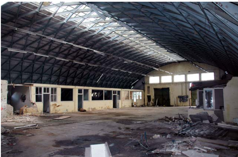
depicted item: inside the Lamella Roof Hall source: Andreas Butter date: 2007
