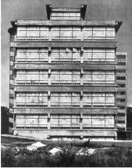
5. depicted item: elevation with possibility of annexation (south elevation) source: Moderne Bauformen 1932, vol. 18, p. 491-499 (Ernst Scheel) date: ca. 1930
