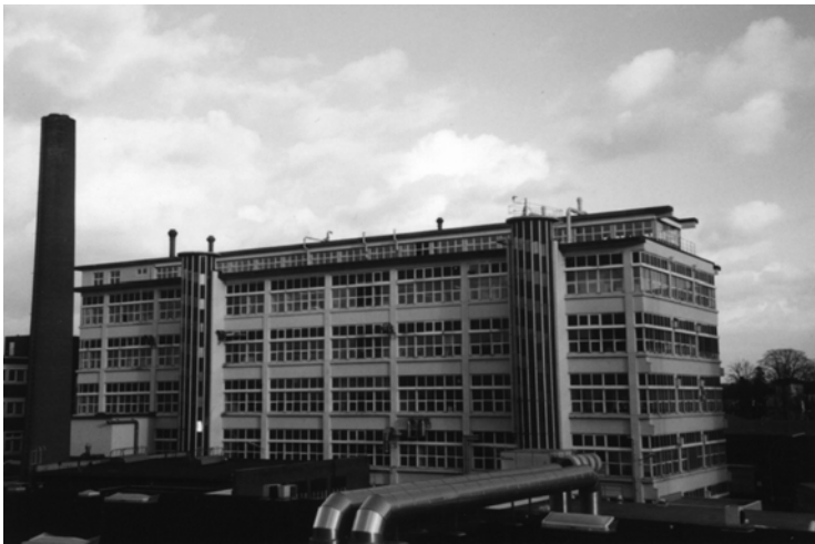
8. depicted item: current condition (west elevation) source: Ingrid Ostermann date: 12/2001
